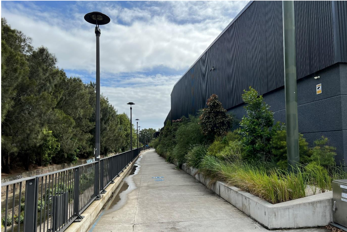
Figure 7: Existing pedestrian/cyclist path along the Shea's Creek channel north of the Huntley Street bridge, connecting to Maddox Street
